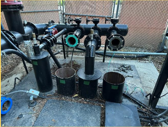
Two pumps being replaced - June 23rd
